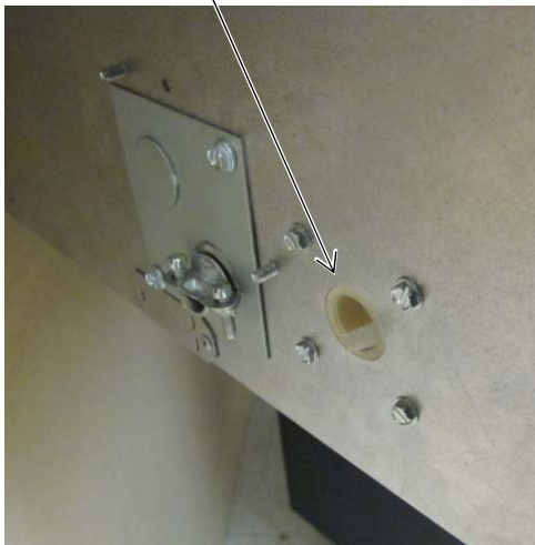
Left Side Gas Line Location
