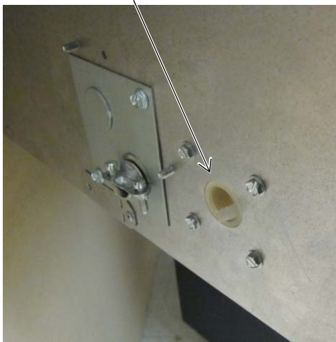
Left Side Gas Line Location
