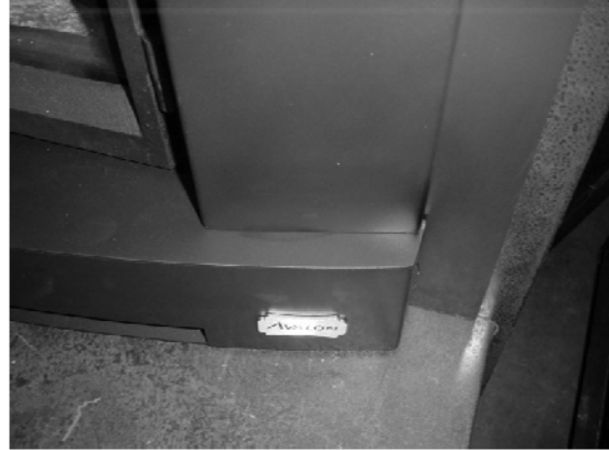
Figure 18: Face aligned flush with the insert
