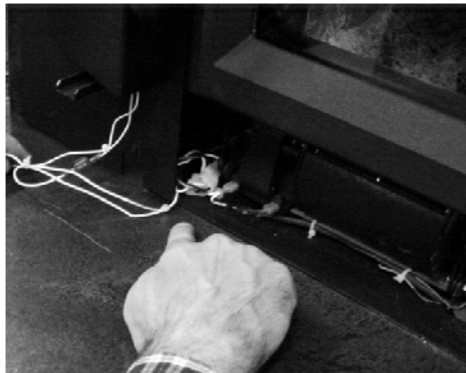
Figure 11: Tuck excess wires
