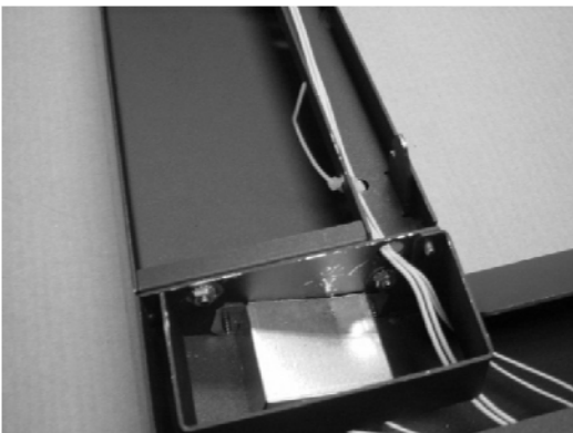
Figure 7: Wires secured with lock-tie
