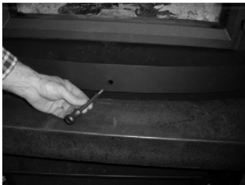
Figure 21: Attaching the air control rod
