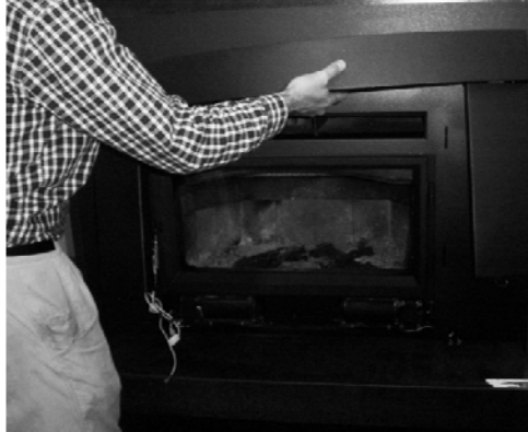
Figure 9: Attaching the face
