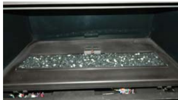
1) Start installing Crystals on the Burner
