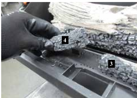
Log 4 rests against tab on burner
