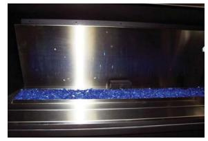
2) Install a side panel next (not important which side goes in first). Position the panel with the bend in the panel facing towards the outside or wall of the unit. Position side panel and secure with a clip and one screw.  Install other side panel next. Position side panel and secure with a clip and one screw.
