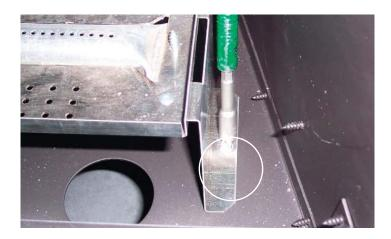
12) Slide the burner to the right and lift up and out of the firebox.
