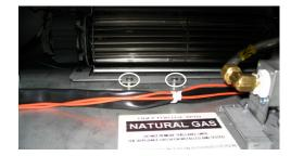
9) Carefully slide the fan to the front, rotate it 45 degrees and slide it out simultaneously with the ECS box.
