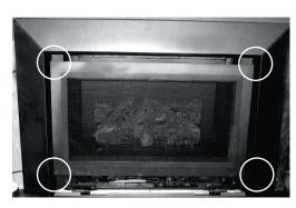
Note: Ensure that the flanges on the sides of the firebox are on the outside, when installing the faceplate (see below).
