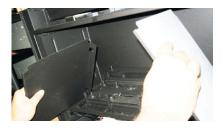
Orient the stainless side panels with the larger fold in the panel facing in towards the burner and facing the back of the firebox
