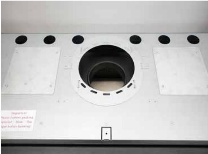
1. 6" starter flue fitted. Note the crimped end is down (into unit)
