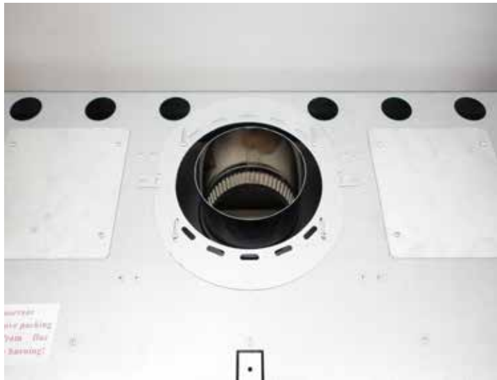
2. 6" Flue fitted. Note: crimped end is down. Must connect active pipe using stainless steel rivets or self drilling screws. 2 for each join..
