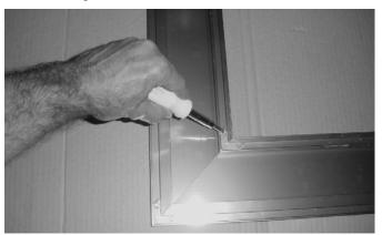
11 Hang the trim on the brackets as shown below. The lower brackets, with magnets, will attach the lower part of the trim to the face. Make sure the trim is centered on the fireplace.
